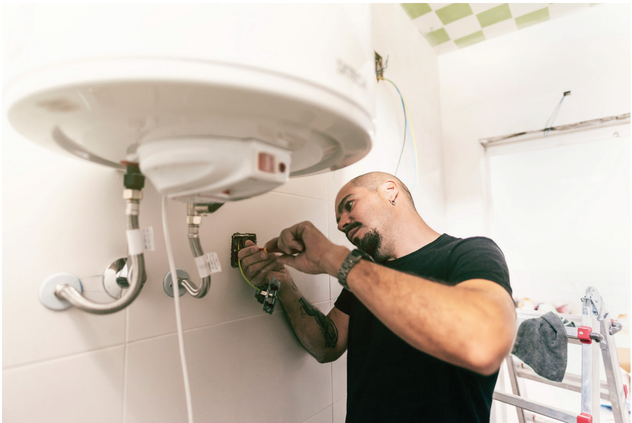
An electrician installs an electric hot water heater. Getty Images
