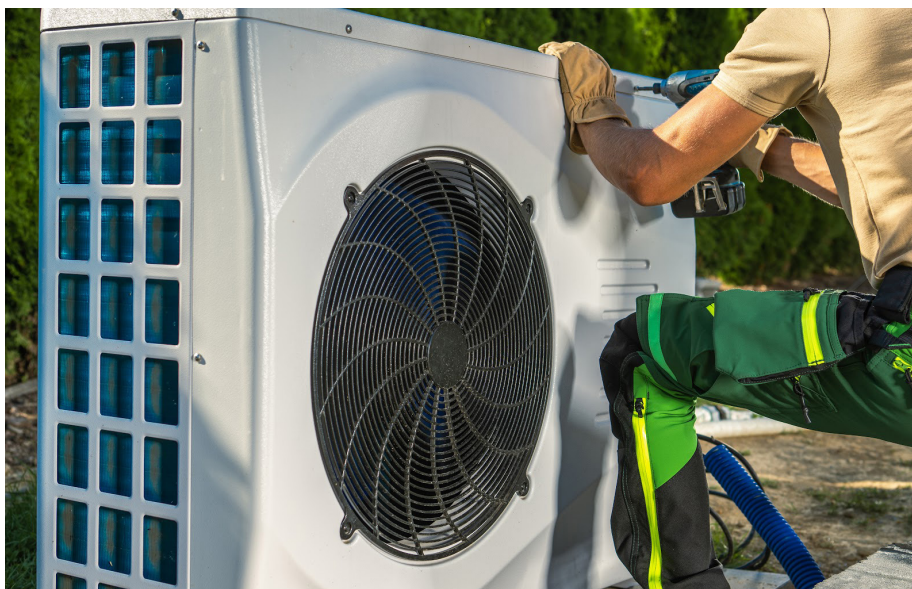
Source: Getty images An HVAC worker installs a heat pump
